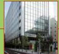
Japan Distribution Center
