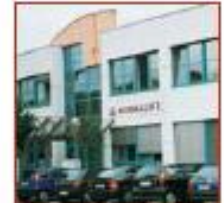
Germany Distribution Center
