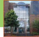
U.K. Distribution Center
